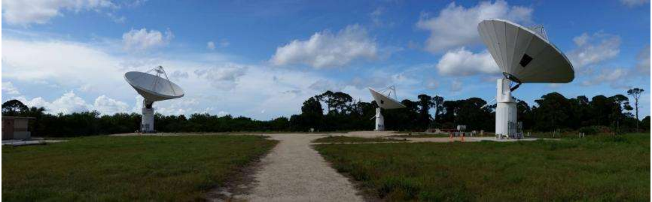
Figure 14. KaBOOM antennas at KSC.
