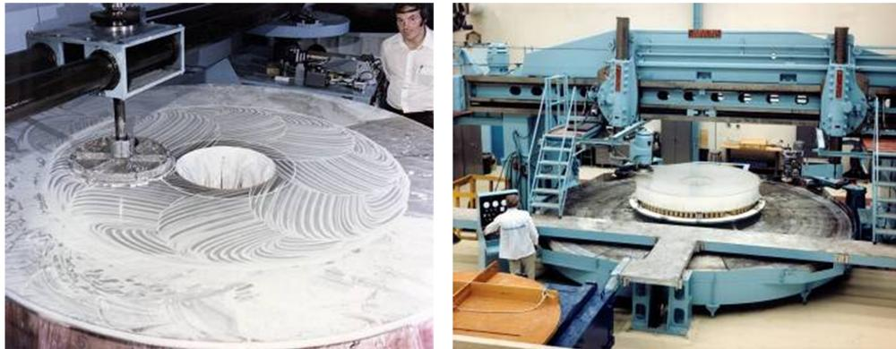
**Fig. 19** Hubble primary mirror fabrication 1979–1981 (courtesy Goodrich).
